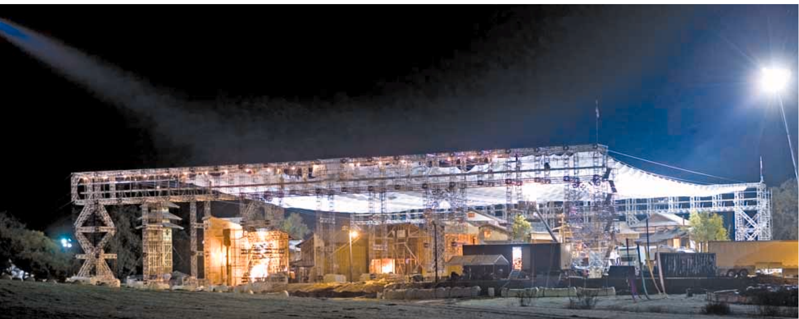
A nighttime view of the truss rigs. Measuring 50' high x 260' long, the structures stood 300' apart.
